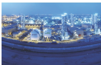
Completed Phase II of Jazan Gasification and Power Joint Venture
