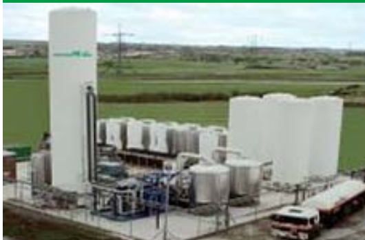
Onsite Gas Supply
